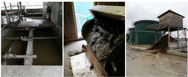
Figure 1Separate production by pumping and pressing manure
